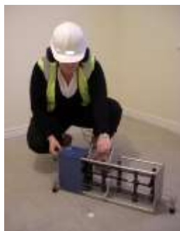
Figure 4 Impact sound test being carried out
